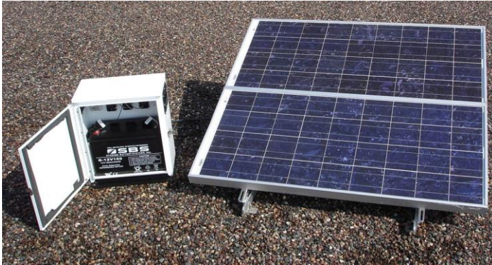
Figure 10: Solar power system (854060)
