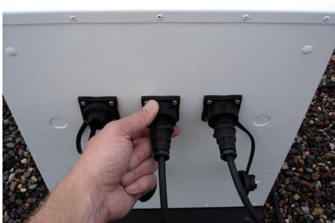
Figure 39: Connect Solar Cells to Battery Enclosure Box
