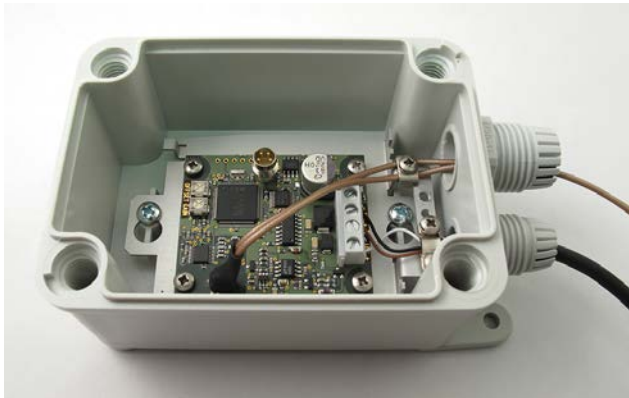
Figure 5 Bracket Installed and Cables Connected
