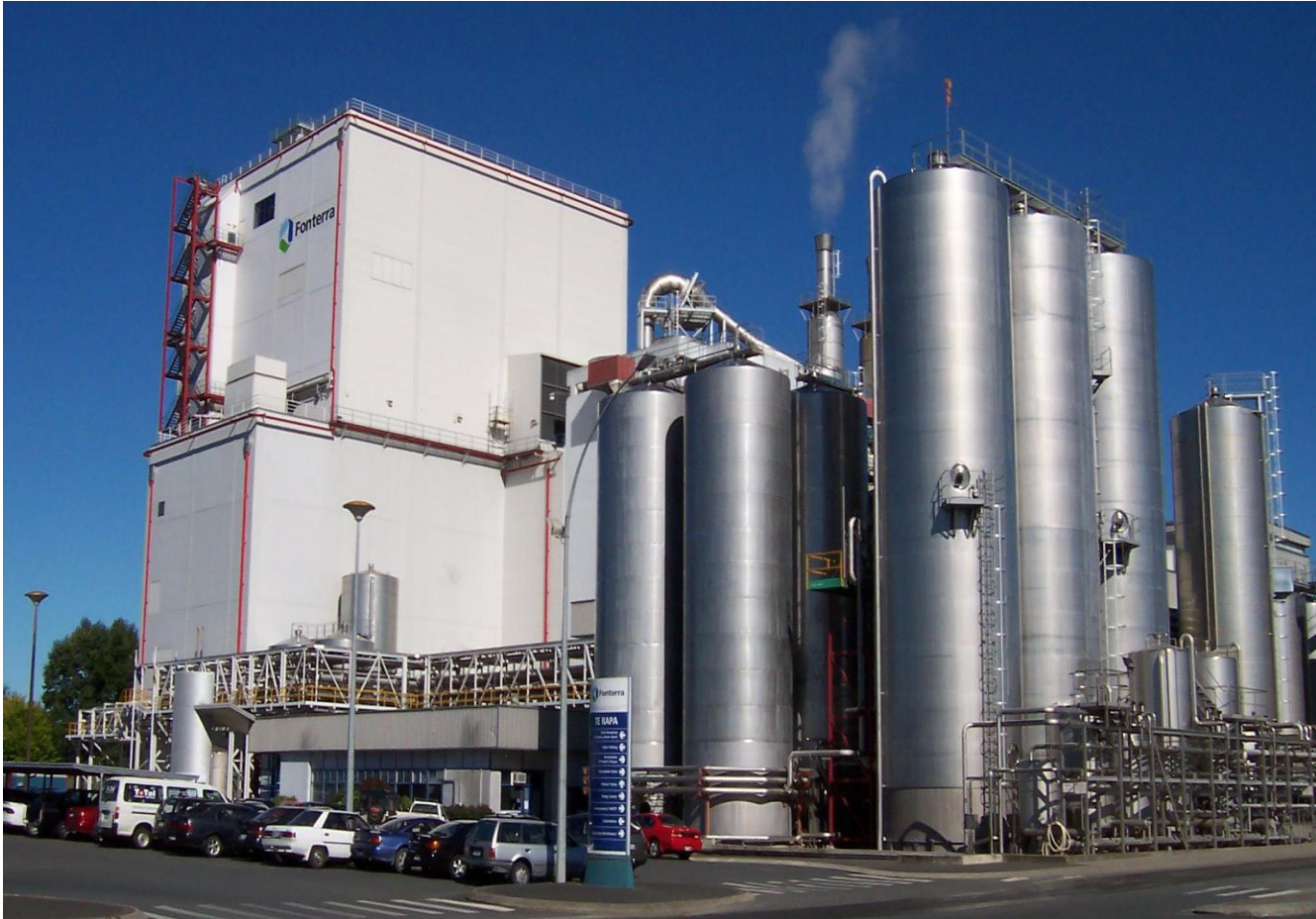
Fonterra Dairy Factory-Te Rapa, New Zealand
